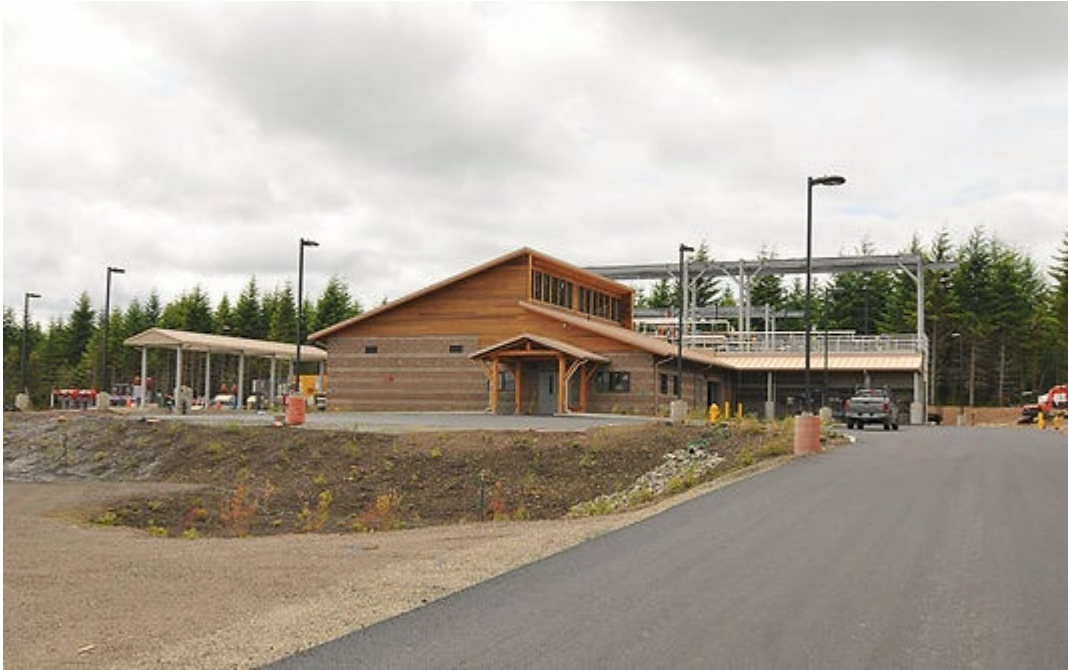
Belfair Wastewater and Water Reclamation Facility (WWRF). Source: Boss Construction, accessed 2026.
