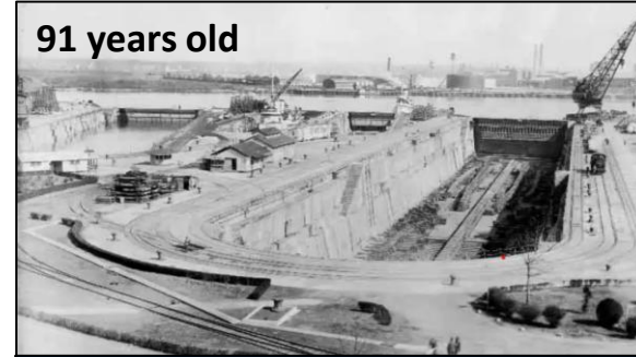
NNSY Dry Dock 3 (ca. 1935)
