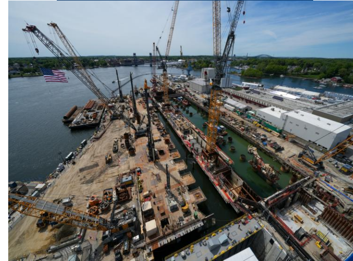
PNSY Dry Dock 1 Expansion
