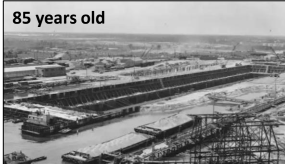
NNSY Dry Dock 8 (ca. 1941)
