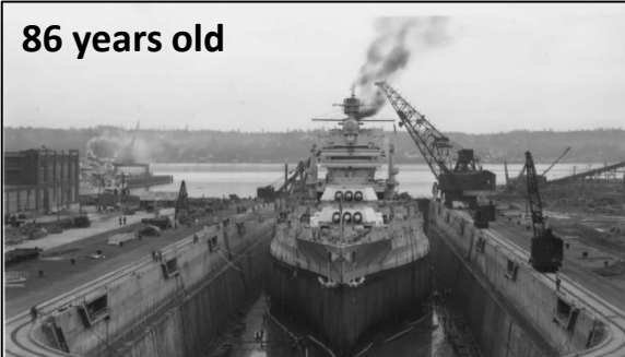
PSNS Dry Dock 4 (ca. 1940)
