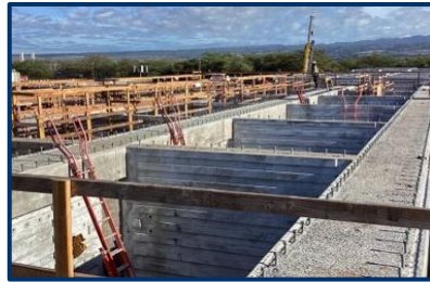
PHNSY DD5 Floor Unit Fabrication
