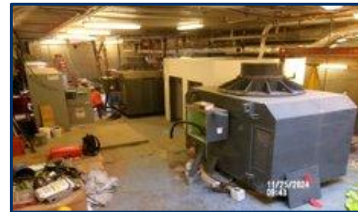
NNSY DD8 Pump Well Motor Install
